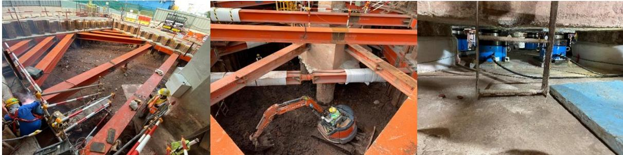
Figure 5. Images of underpinning works at pier FP9
