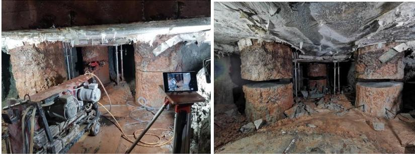
Figure 13. Images of the piles during (left) and after (right) the pile cutting
