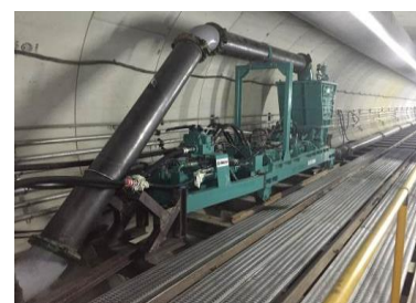
Figure 5. Telescopic Snake (left) and PE booster pump (right) (from Route 479 Shimizu Utility Corridor Tunnel, Osaka, Japan)
