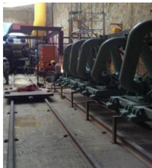
Figure 6. Muckpump Hopper (left) and Snake Pipe Extension (right) on Thomson Line C925
