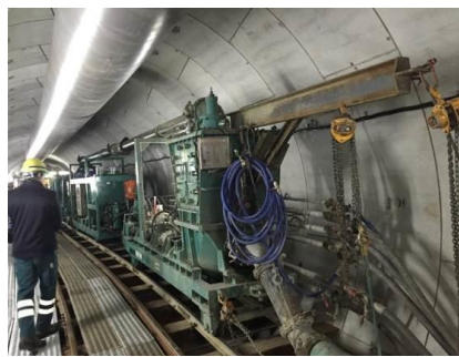
Figure 4. P0 Primary Pump and P1 Secondary Pump (from Route 479 Shimizu Utility Corridor Tunnel, Osaka, Japan)
