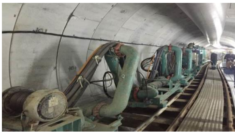
Figure 5. Telescopic Snake (left) and PE booster pump (right) (from Route 479 Shimizu Utility Corridor Tunnel, Osaka, Japan)
