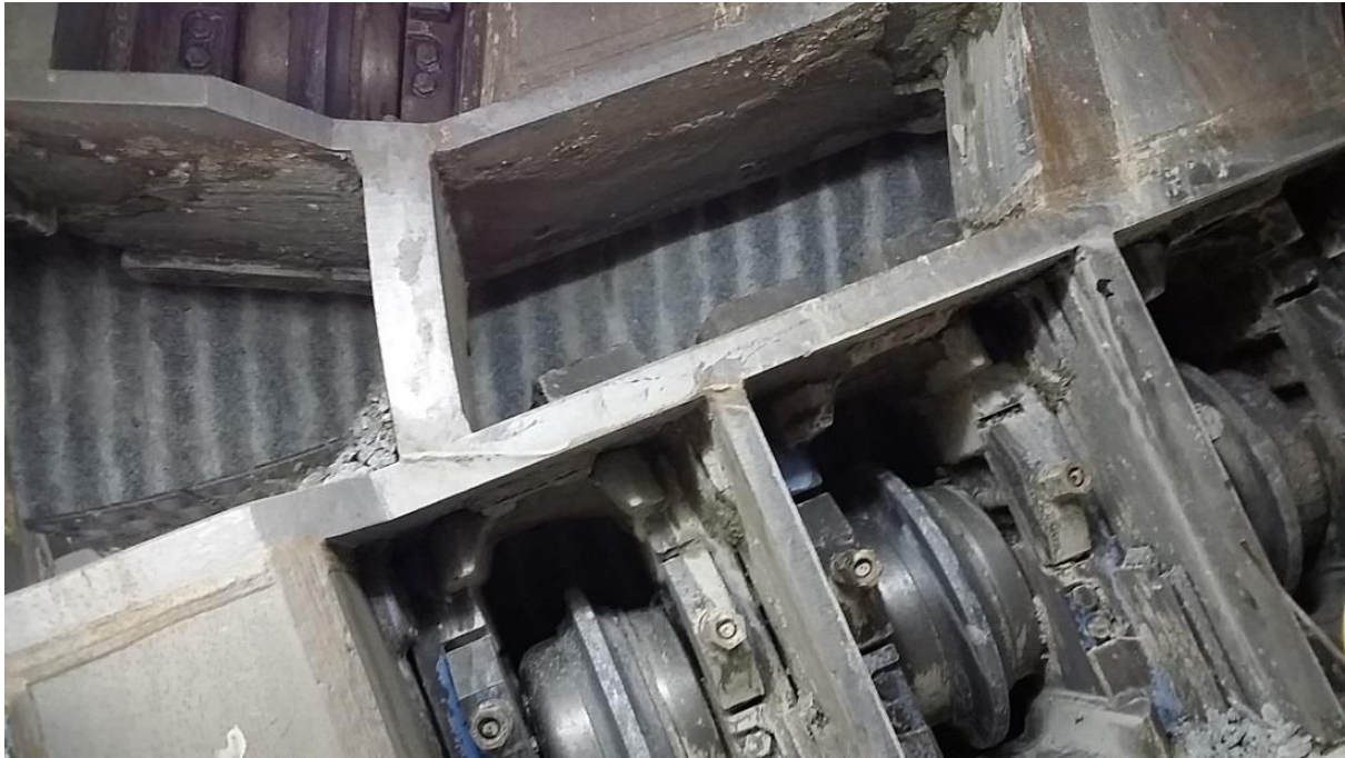
Figure 3 - Photo of free air intervention in intact BTG rock, showing stable and dry condition at the face.
