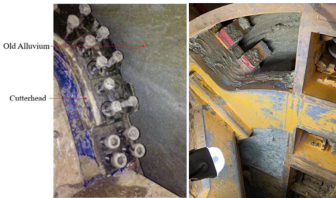
Figure 4 - Photo of free air CHI in competent ground (OA).
