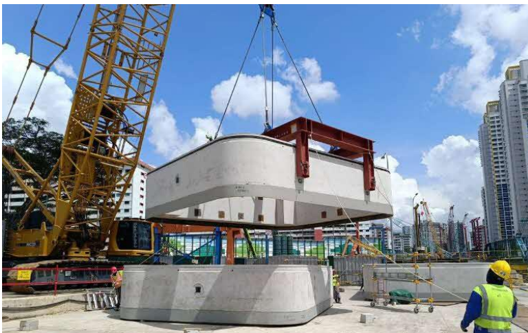
Figure 17. Shifting of Segment using Spread Beam
