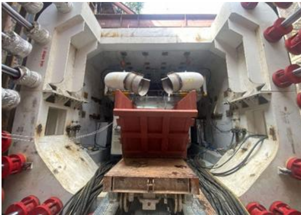
Figure 5. RPJM Double Screw Conveyor System for controlled muck disposal
