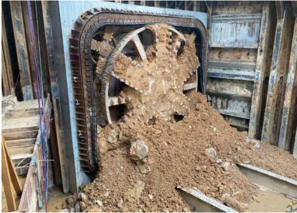
Figure 13. RPJM Breakthrough at Entrance 4
