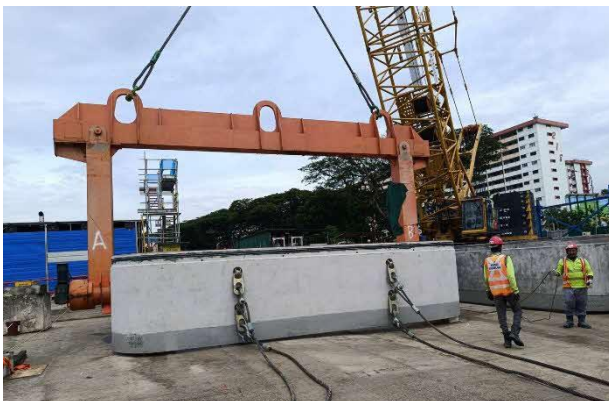
Figure 19. Lifting Lug and Wire Rope attached to the segment
