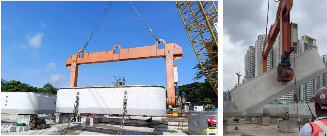
Figure 18. Turning of Segment from Horizontal to Vertical
