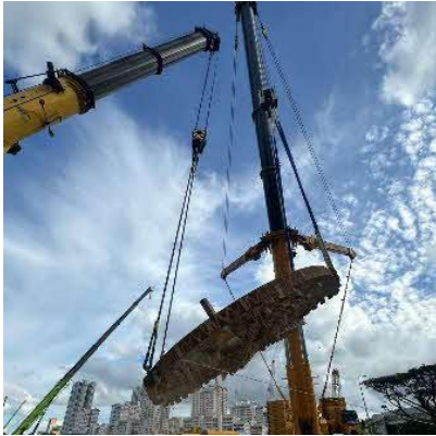
Figure 15. Tandem Lifting
