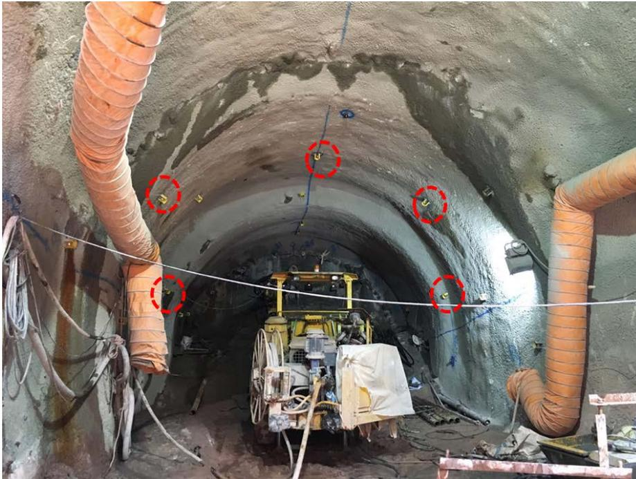
Figure 3: Location of 3D prisms in the mined tunnel
