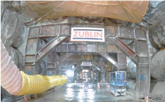
Figure 13: Temporary steel frame
