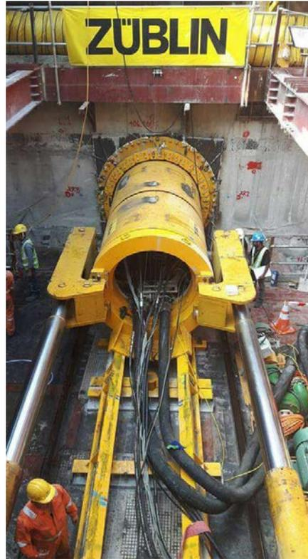
Figure 9: Pipe Jacking Setup
