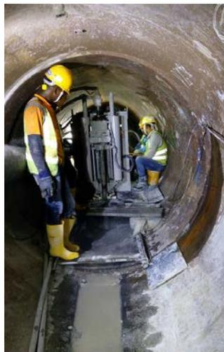
Figure 12:JGP rig in limited headroom condition (inside roof pipe)
