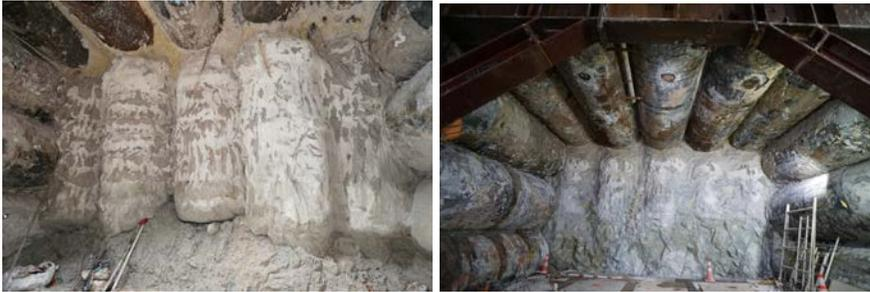
Figure 11: Jet Grout Piles – Visible during excavation of tunnel
